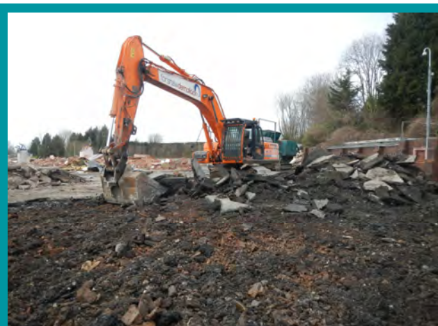
Hard-standing under removal.
